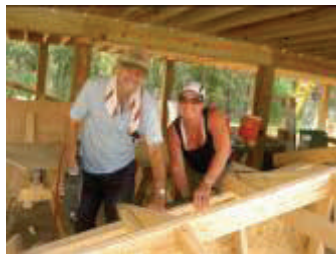
Curtis and Dawn work on a roof dormer.
